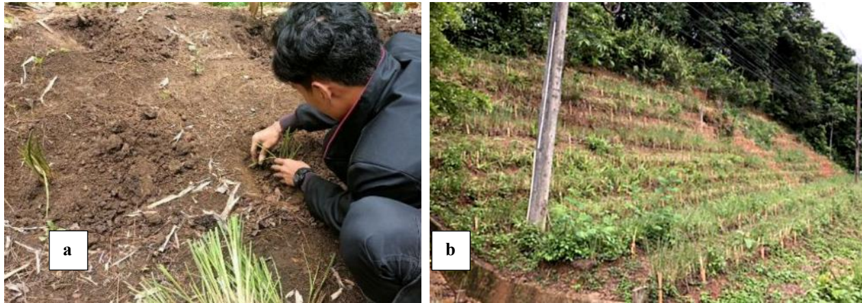
Figure 10. a) Application of Vetiver in Malang, East Java Indonesia (Rahayu & Hidayat, 2025) and b) Huai Khayeng Area, Thailand (Leknoi & Likitlersuang, 2020).
